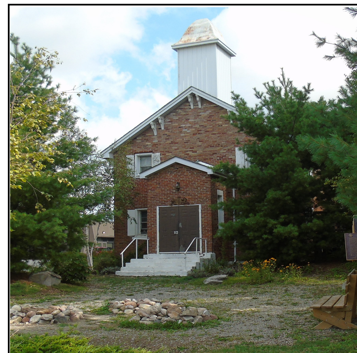
New Credit Council House
